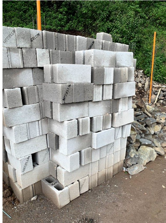
Photo 7: CMU used in the construction of residential house.
